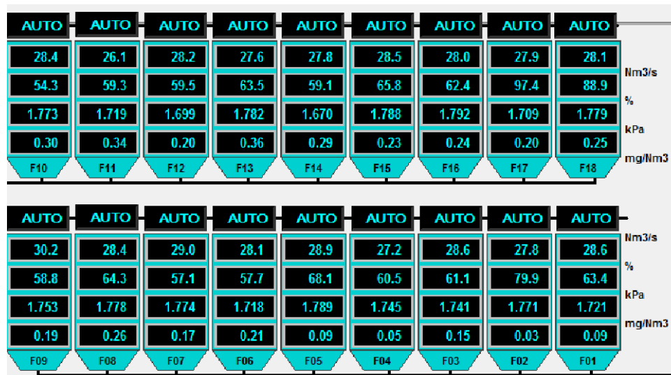
Figure 13. An HMI view of filter parameter in GTC.
